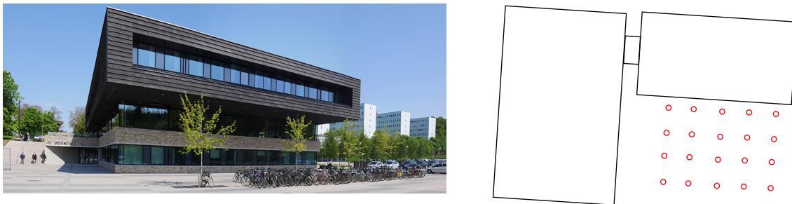
Fig. 1. Studenthuset in Stockholm, front view (left) and top view with borehole field (right). Photo: Jeffrey D. Spitler.
