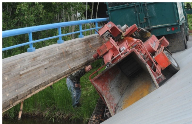
Figure 1: North Westchester Lagoon Bridge
