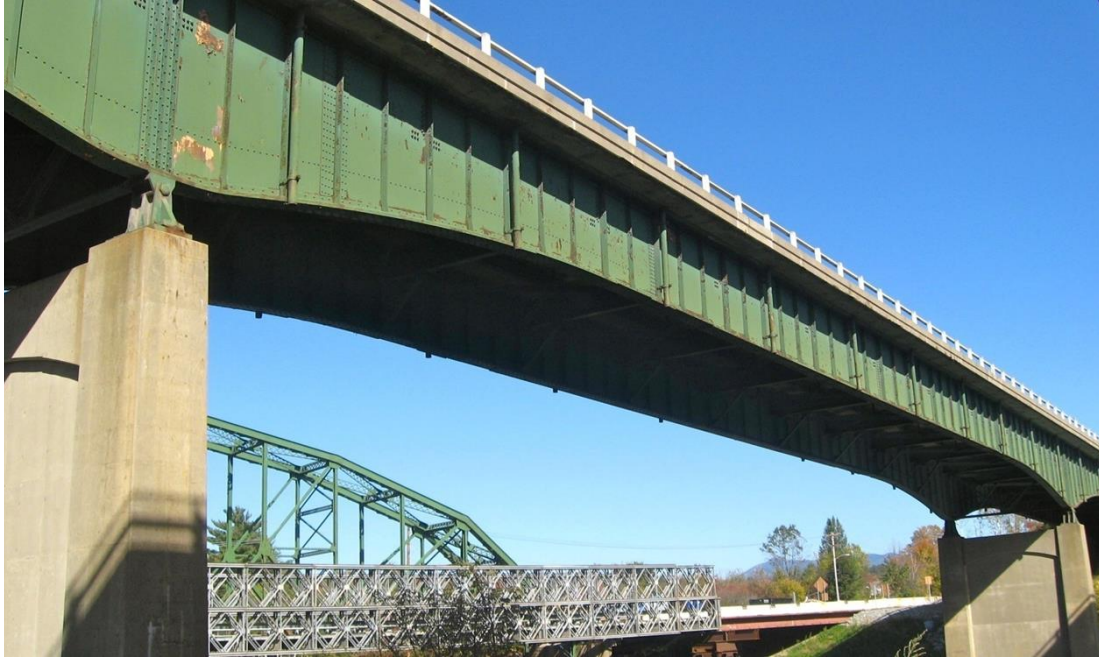
Figure 4.9: Photograph of bridge 58N located in Vermont, USA.
