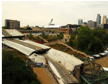
(b) After collapse
