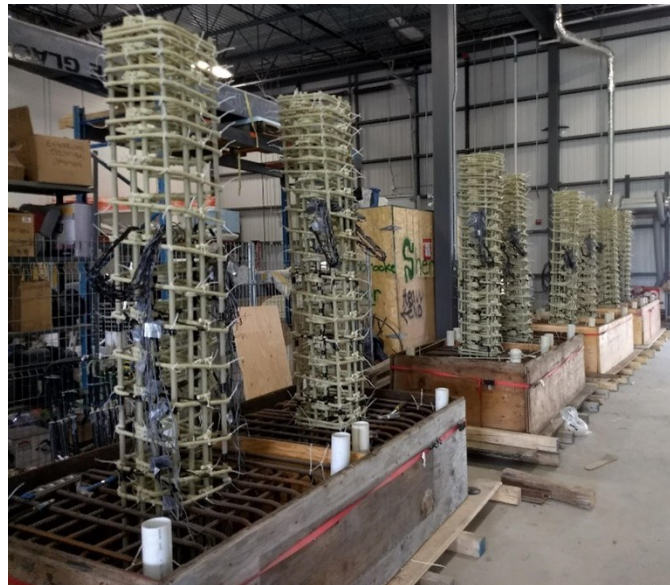
Figure 3.10- Placing column inside the stub steel cage
