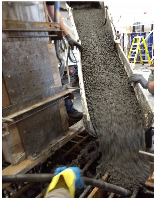
Figure 3.12- Casting of stub
