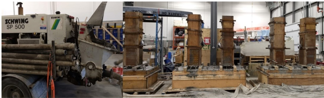
Figure 3.13- Casting of column
