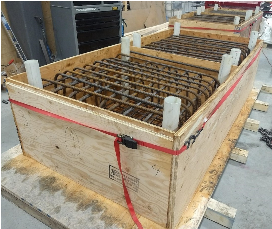
Figure 3.6- Placed PVC pipes and stub steel caging
