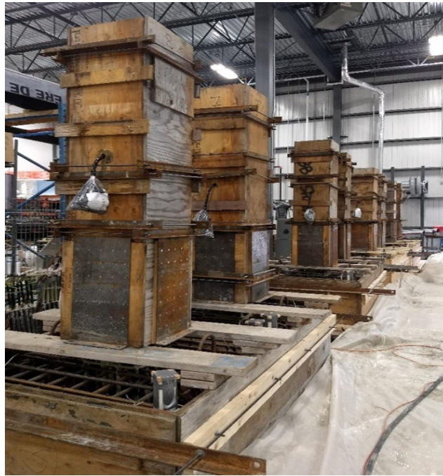
Figure 3.11- Covering the column cage with formwork.
