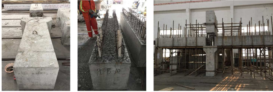
(a) PC columns (b) PC beams (c) Assembly construction
