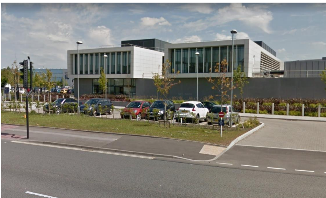
Figure 2: Patchway Police Station. Source: Google maps
