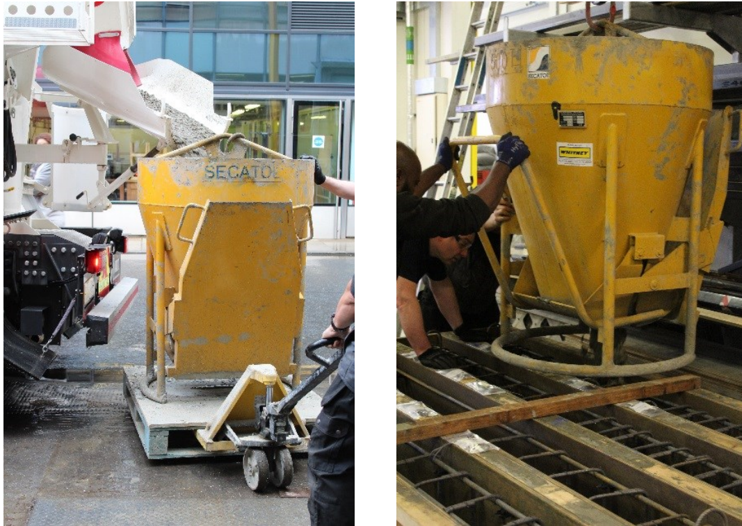
Figure 3.8: Pouring of the concrete
