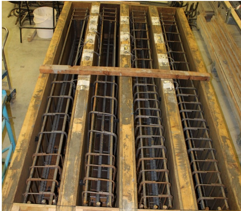
Figure 3.7: Reinforcement cages inside the moulds before casting.
