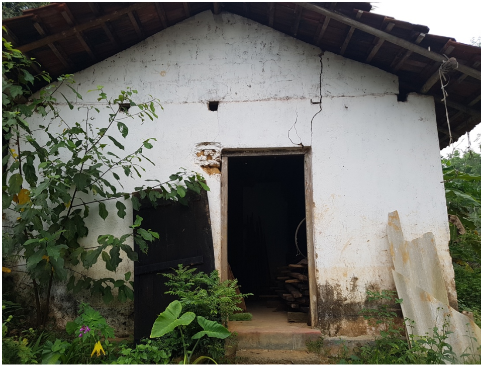
Figure 4. Cracking around opening
