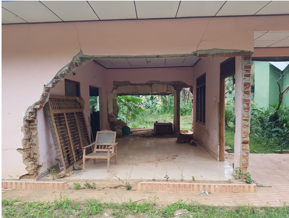
Figure 1. Flood damaged masonry house, Sri Lanka, 2017
