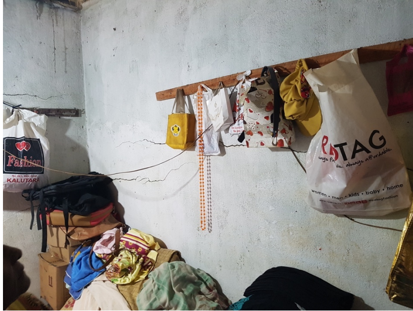
Figure 3. Cracking in solid wall
