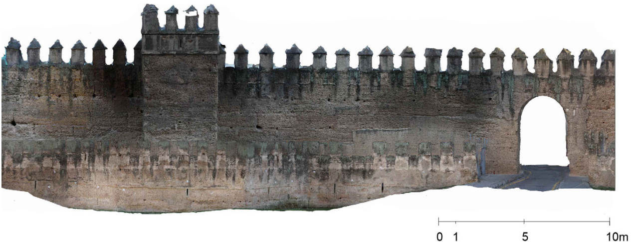
Fig. 14. Orthophoto of the principal view (Source: the authors).
