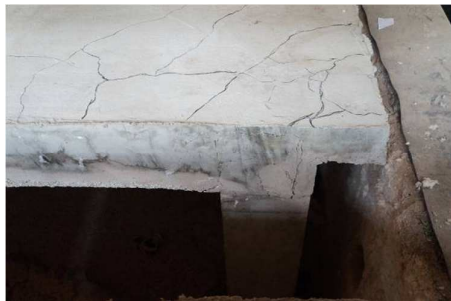
(j) Beam-column connection in Test 2 (North-east corner)
