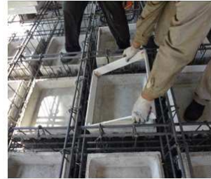
(i) Installation photo for the side wall of the assembly box
