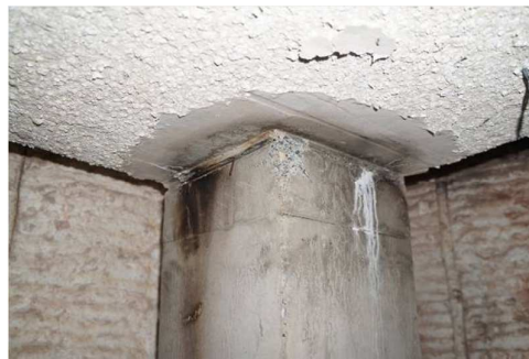
(h) North-east corner column in Test 2
