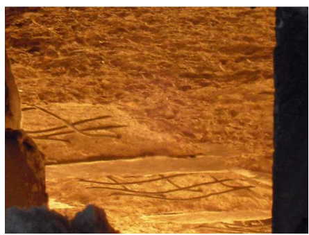
(a) Concrete spalling of the bottom plate
