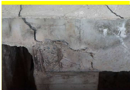
(i) Beam-column connection in Test 2 (South-east corner)
