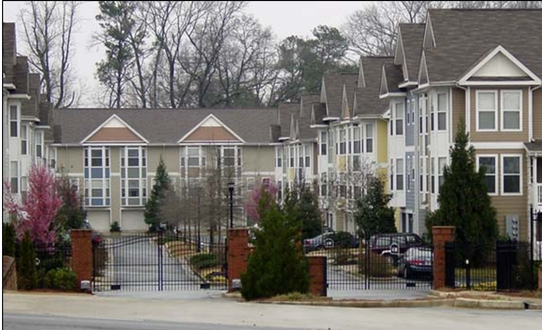
Figure 34 Adaptation of New Urbanism: Glenwood Green, Georgia
