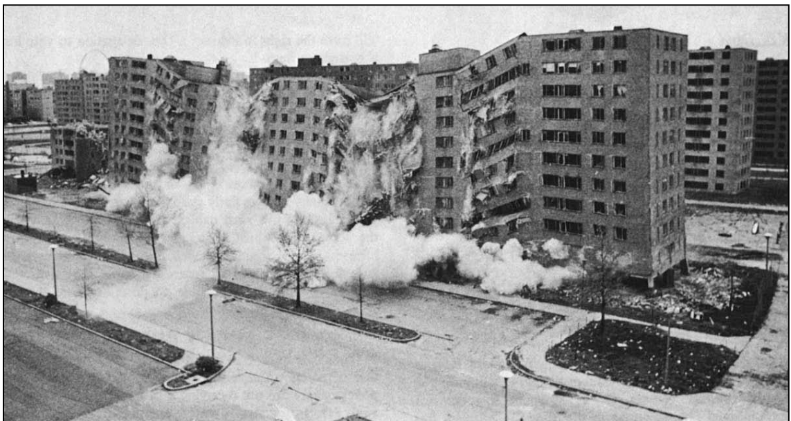
Figure 24 Demolition of Pruitt-Igoe Complex in St. Louis, Missouri (Source: Wikimedia Common 15 )
