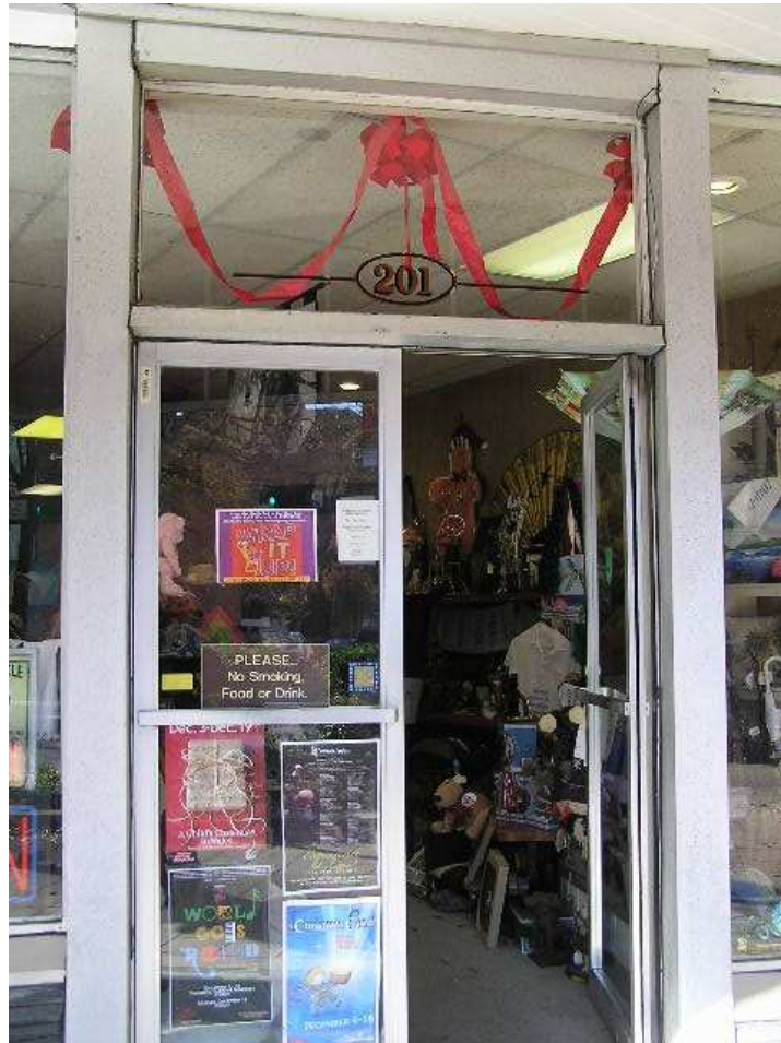
Figure A.3 Photograph of a small shop in downtown Greenville.
