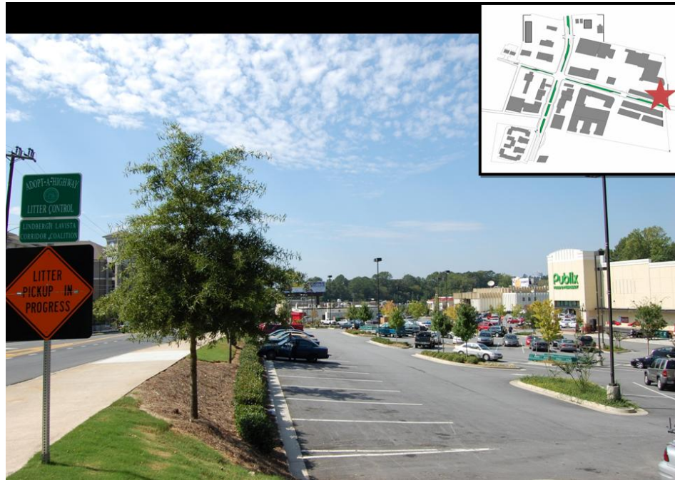
Figure 4.2-27: Current surface parking.
