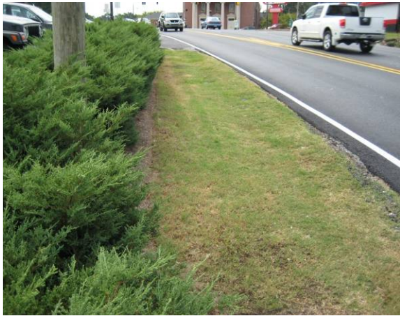
Figure 2.2-8: Some of the sidewalks in the study area are located too close to the road and lack a buffer for safety and ease of mind.
