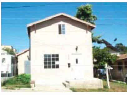
Vacant property before and after rehabilitation
