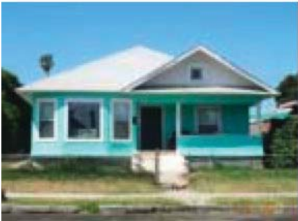
Vacant property before and after owner rehabilitation
