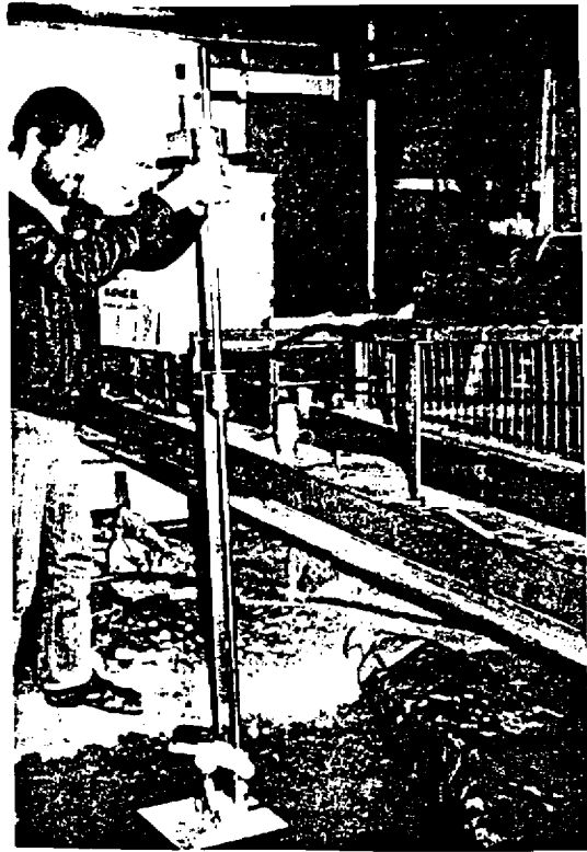
Figure 35. Dynamic Cone Penetrometer Test on Subgrade.
