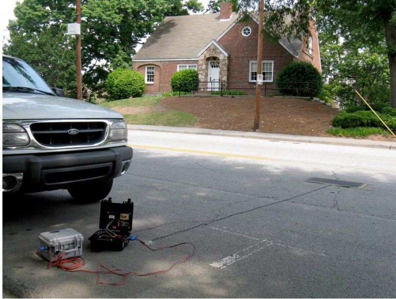
Figure 30 - Fifth Field Test, 5/14/2010, Along Eastbound Ferst Drive
