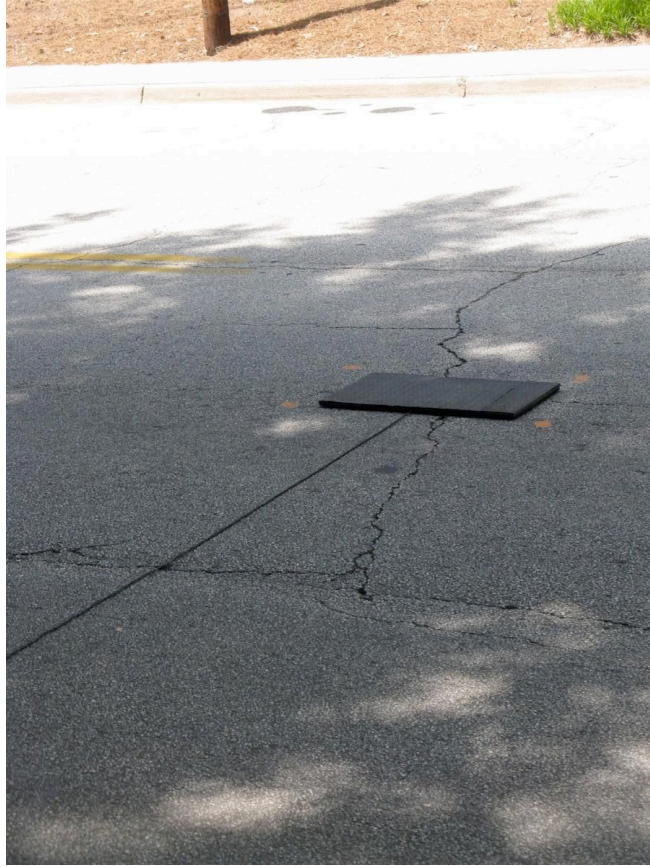
Figure 46 - Intermediate Size Loop Deployed Longitudinal to Traffic, During Seventh Field Test
