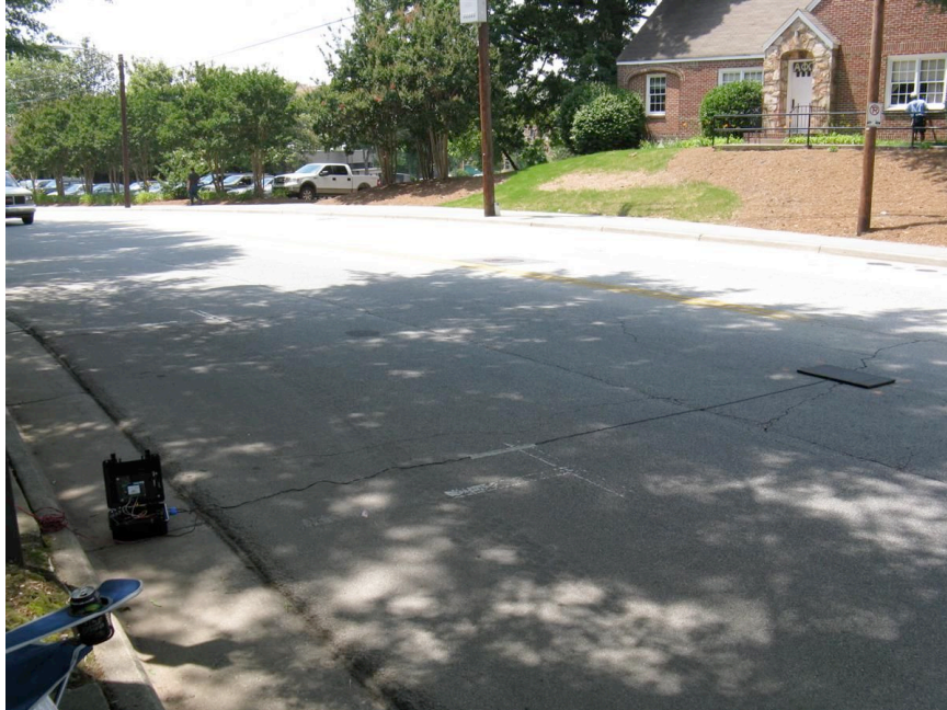
Figure 45 - Test Site on Eastbound Ferst Drive with Intermediate-Size Loop Mounted Longitudinal
