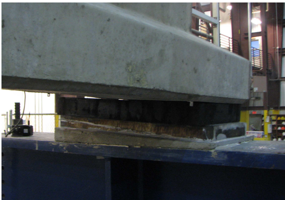
(a) East End Support before Retrofit
