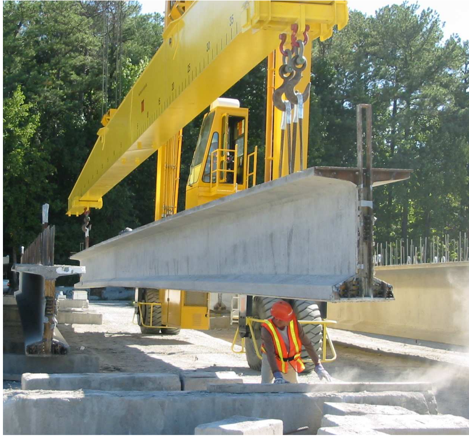
Figure 2.6 – Completed fabrication of BT-54 girder
