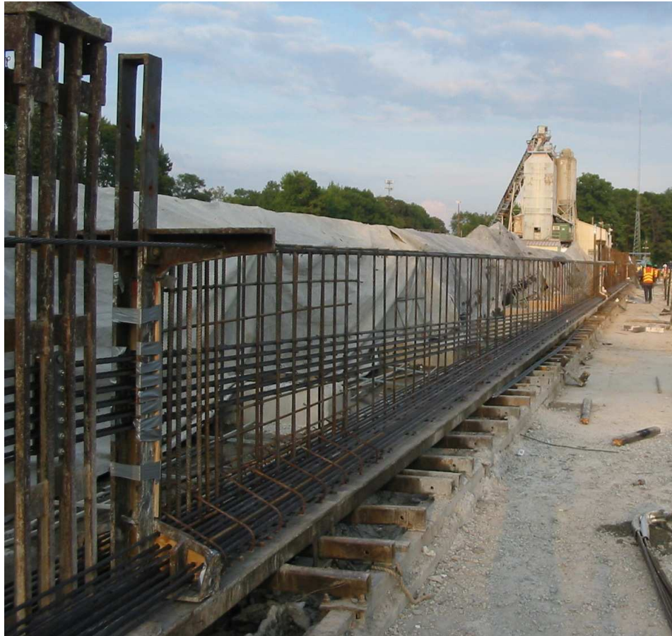
Figure 2.5 – BT-54 girder during fabrication
