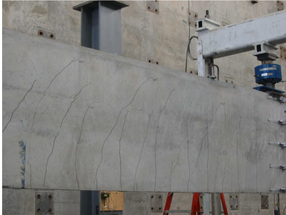
Figure 5.68 – Photo of diagonal cracking at the buckling load for Beam C2B
