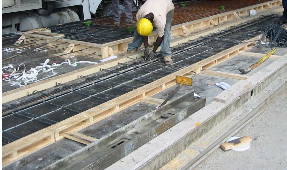
Figure 2.2 – Reinforcement placement during fabrication of rectangular beams
