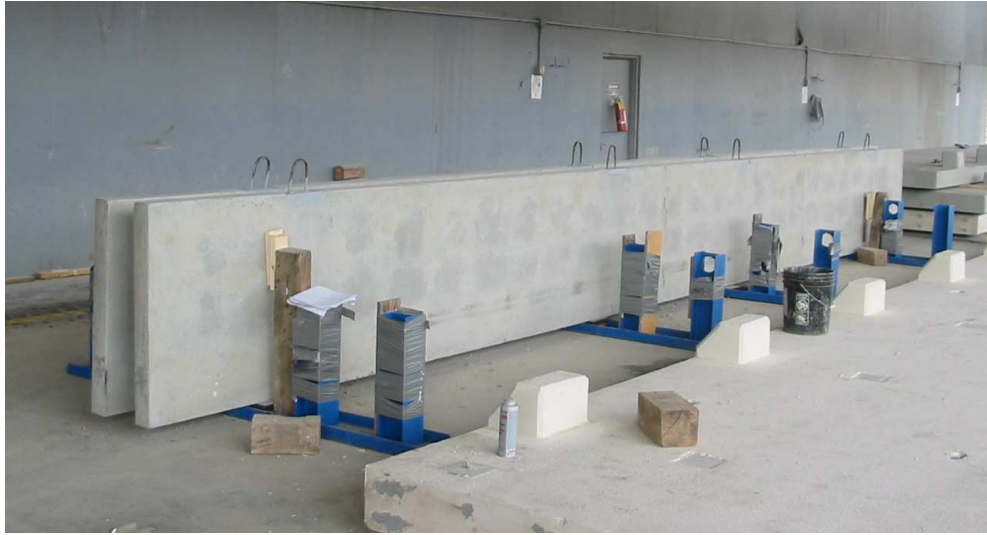
Figure 2.3 – Finished rectangular beams
