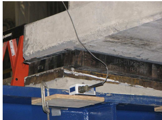
(b) East End Support after Retrofit
