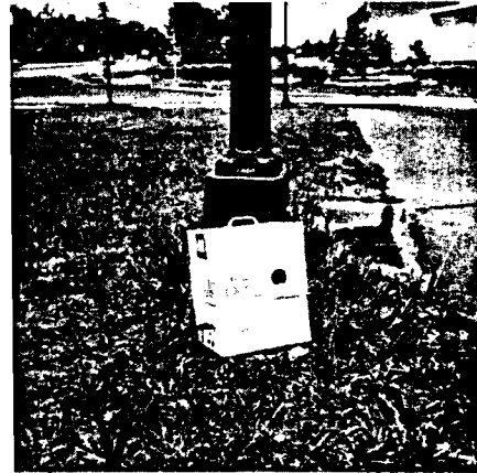
Figure 2. The wrong-way camera unit, installed and chained to light standard
