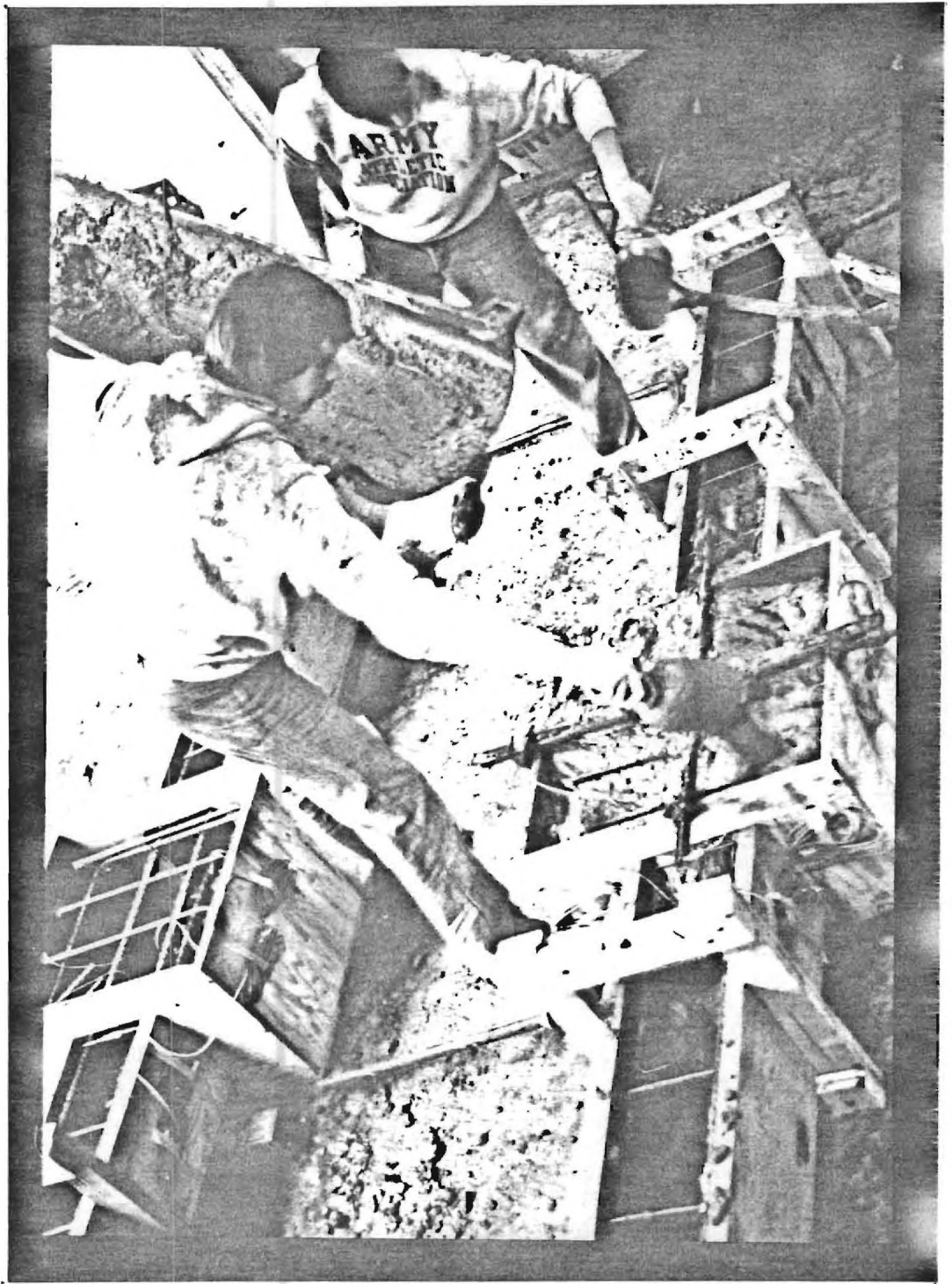
Figure 3. Casting columns in horizontal position with ready-mix concrete.
