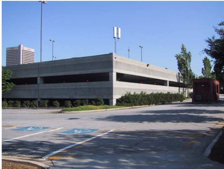
Figure 3.11 East side of Student Center Parking Deck (medium-tier base station on utility pole on the corner of the structure.)
