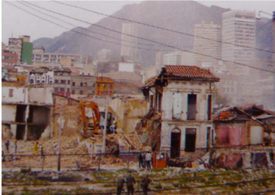
Demolition of Cartucho – Copyright reserved – Source Internet
