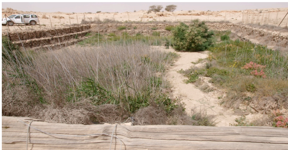
Figure 64 Tiered walls and dam at the base of a depression, fed by a number of inlets
