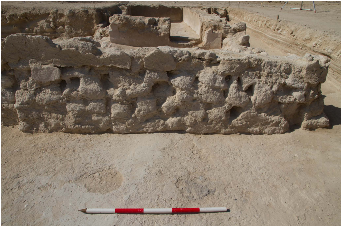
Figure 2.8: Postholes interpreted as temporary support posts
