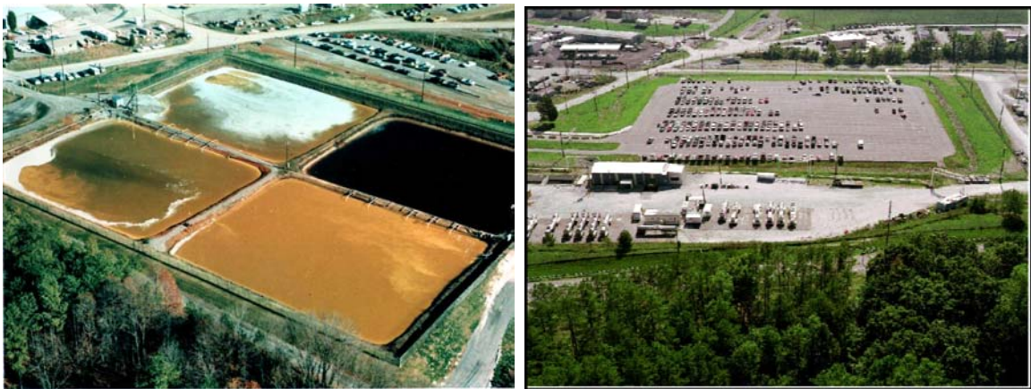
Figure 1.1 The former S-3 Waste Disposal Ponds located near the Oak Ridge Y-12 Plant in Bear Creek Valley (left). The unlined ponds received highly acidic uranium nitrate liquid wastes from 1951 to 1983 (Brooks, 2001). The ponds were capped in 1984 after treatment and removal of liquid wastes (right). Picture from http://public.ornl.gov/orfc/orfc3_site.cfm#Anchor1 .
