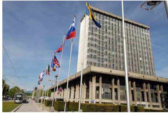
Figure 3. Grenoble city hall, France.
