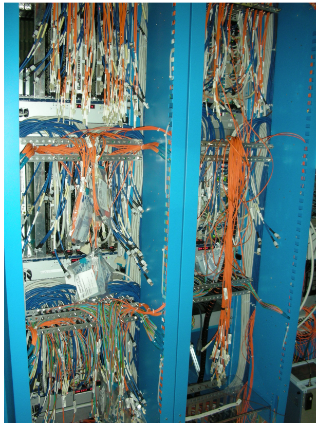
Figure 31. Photo of the two leftmost of five TRT Back End racks in the USA15 counting hall. These two racks house the three 9U crates for End Cap C and the two 9U crates for Barrel side C. The next rack in line house the two 6U ATLAS TTC crates and then two more racks for the side A Back End crates. The electrical and optical cable plant obscures most of the electronics.
