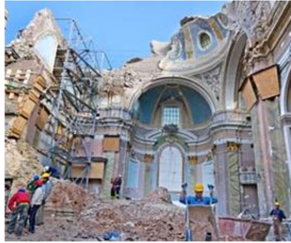
Fig. 4 Observed damage on URM buildings due to intraplate earthquakes after the M6.3 L'Aquila, Italy earthquake occurred in 2009
