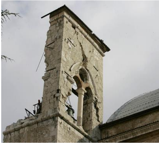
Fig. 4 Observed damage on URM buildings due to intraplate earthquakes after the M6.3 L'Aquila, Italy earthquake occurred in 2009
