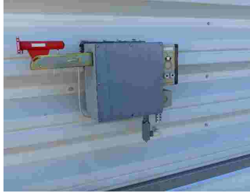
Figure 4.2: Outside Air Weather Station on the Roof of the Klaus Building
