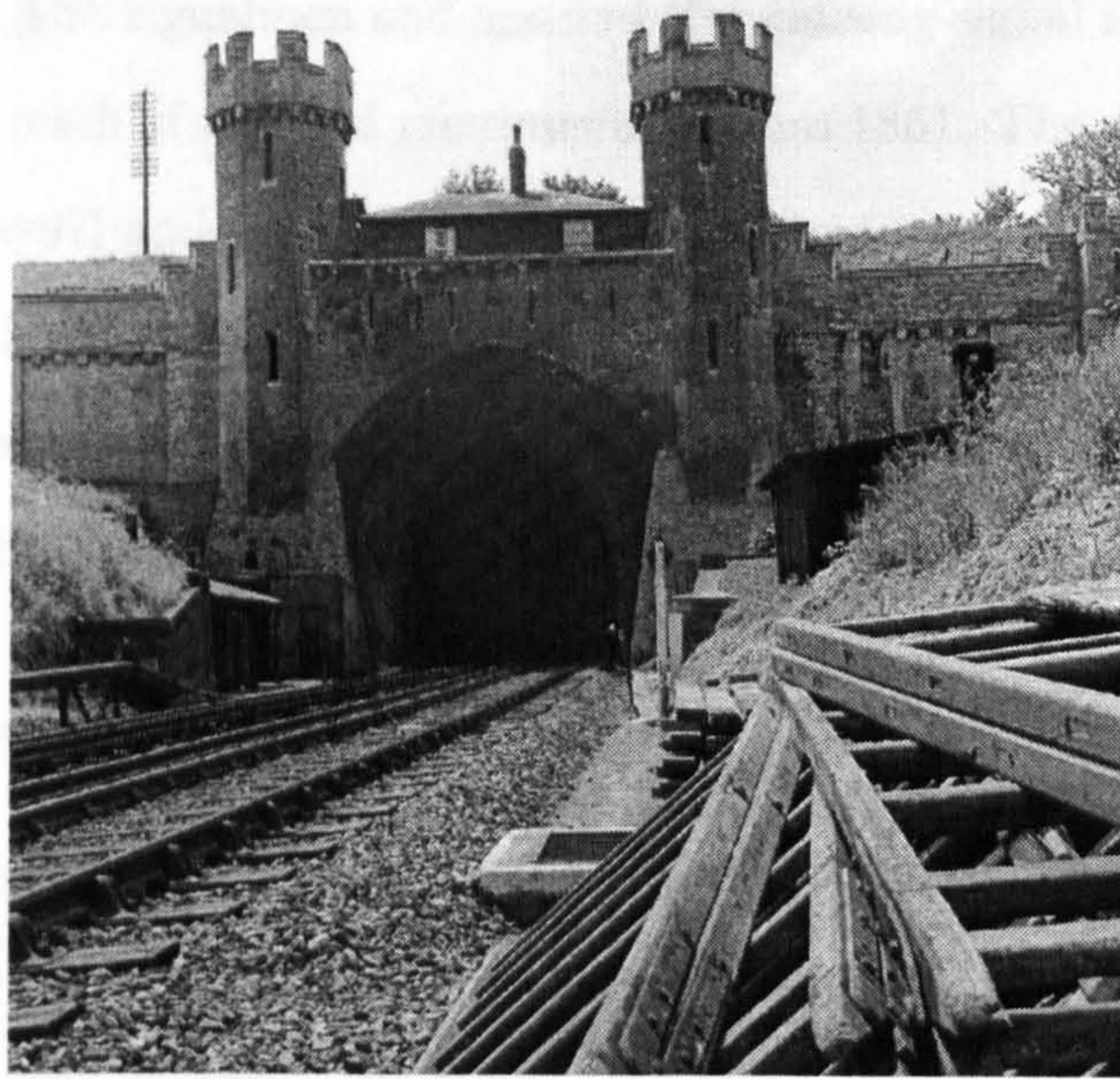
Figure 5.26: A photograph of the Clayton Tunnel (reproduced by permission of English Heritage.NMR).
