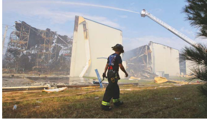
The threat of electrocution from thousands of solar panels on the roof of the Dietz and Watson warehouse in Delano, N.J., slowed efforts to fight a 2013 fire. Photovoltaic arrays are one of many green building features and practices that raise fire safety concerns, research by WPI fire protection engineer Brian Meacham shows. (Photo by the Star-Ledger, Newark, N.J.)
