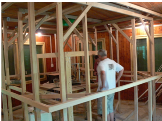
Figure 14. The Braunbek squared coil system in Pruhonice.
