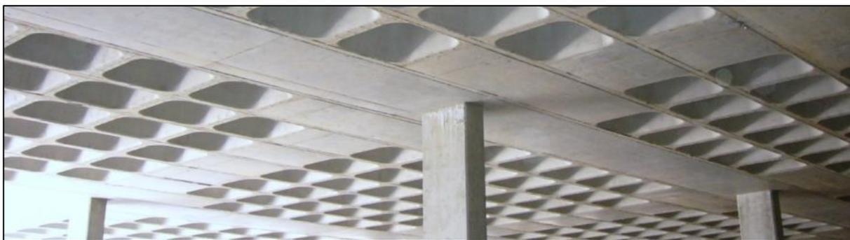
Figura 3.1 – Moldes Ferca - Laje nervurada bidirecional betonada *in situ* [3]
