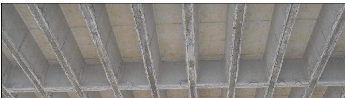
Figura 3.2 – Moldes Ferca - Laje nervurada unidirecional betonada *in situ* [3]
