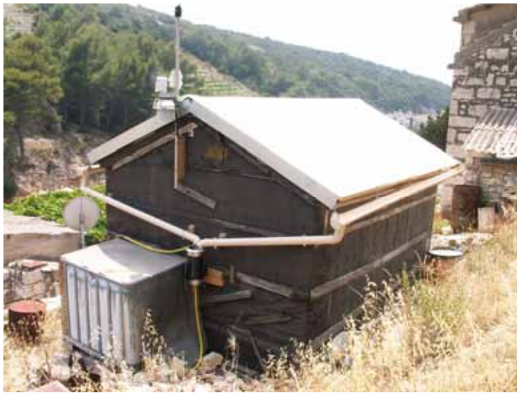
Figure 3. The house in Salbunara bay, NW of Biševo Island. The 15.1 m 2 roof has its symmetry axis oriented east (left)-west (right). Sea is on the west side. (Photo D. Beysens).
