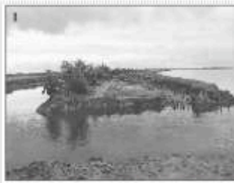
Photo 1 (C. Mazalet, 2003) : brèche accidentelle du polder de Graveyrie (bassin d'Arcachon) / The accidental breach of the sea-dike at Graveyrie Polder (Arcachon Basin, France).
