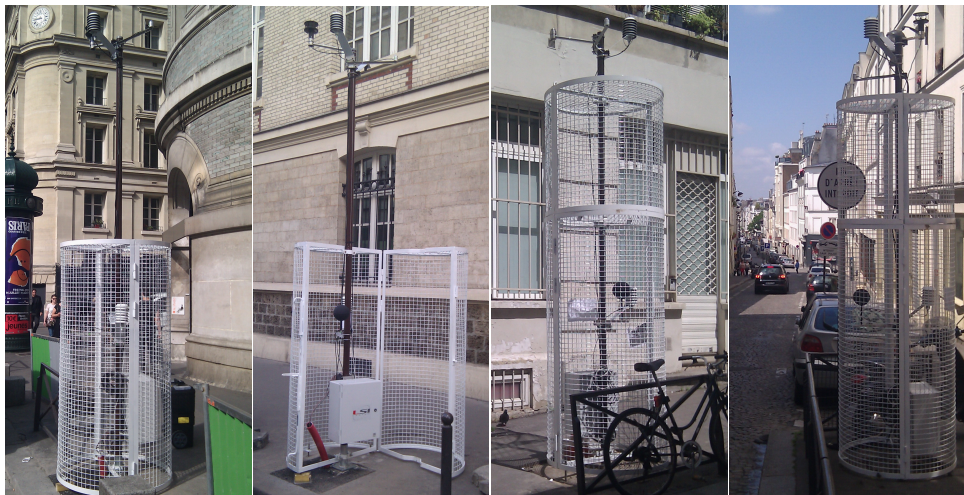
Figure 6.7 – Photographs of watered and control weather stations in situ . From left to right: watered and control Louvre stations, watered and control Belleville stations ( Hendel et al., 2015 ).
