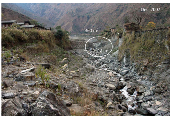
Fig. 2, Ghatte khola, very narrow, undersized hydraulic, cross sectional area of the road bridge, that was destroyed by the monsoon flood in late July 2008 (first season following bridge construction) .
