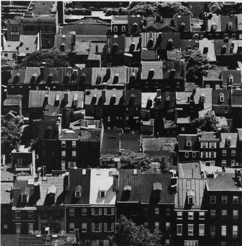
The rooftops of Philadelphia's Society Hill, the site of an intensive renovation program.
