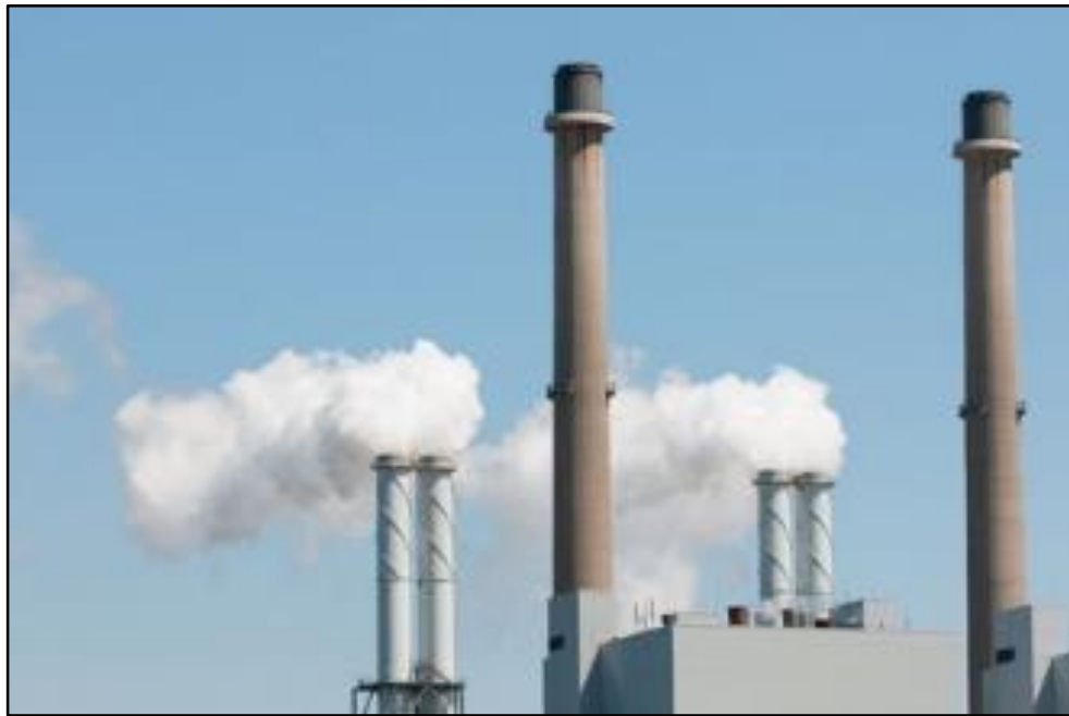
Figure 2: Pollutants pumped into the air from Harding Street plant (Cassell, 2014)
