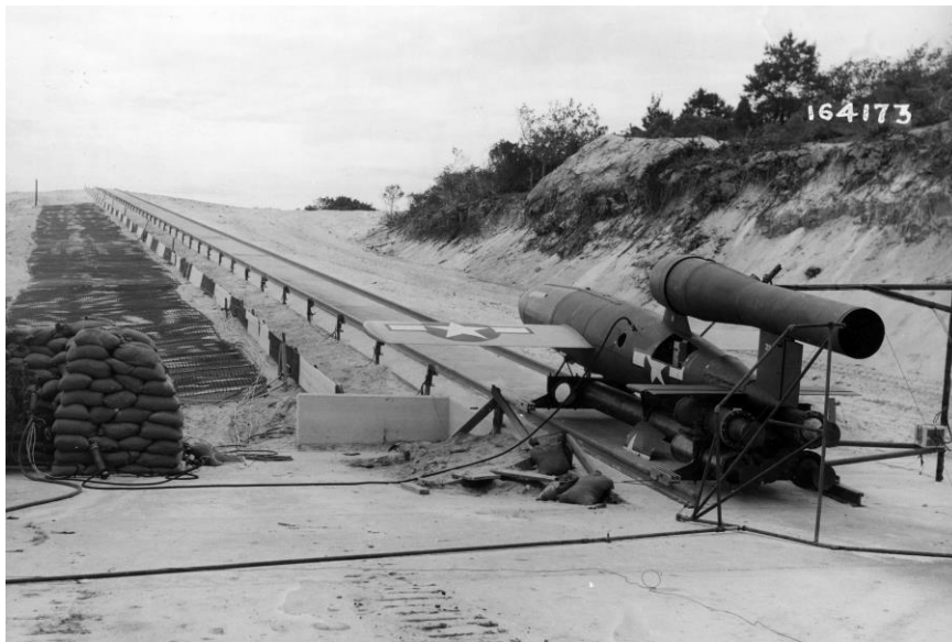
JB-2 on 500-foot, six-degree inclined ramp at Range 64, c.1944. 52
