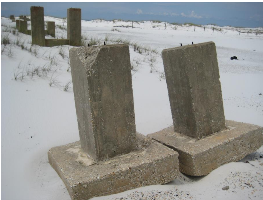
Concrete piers from 400-foot launch ramp at 80K246, June 2012. 169
