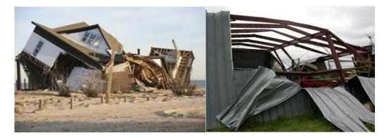
Figure 1.1 Low-rise Industrial Buildings Damaged by High-Wind Events (sources <u>http://www.ARA.gov/</u> and <u>http://www.weather.gov/</u>)
