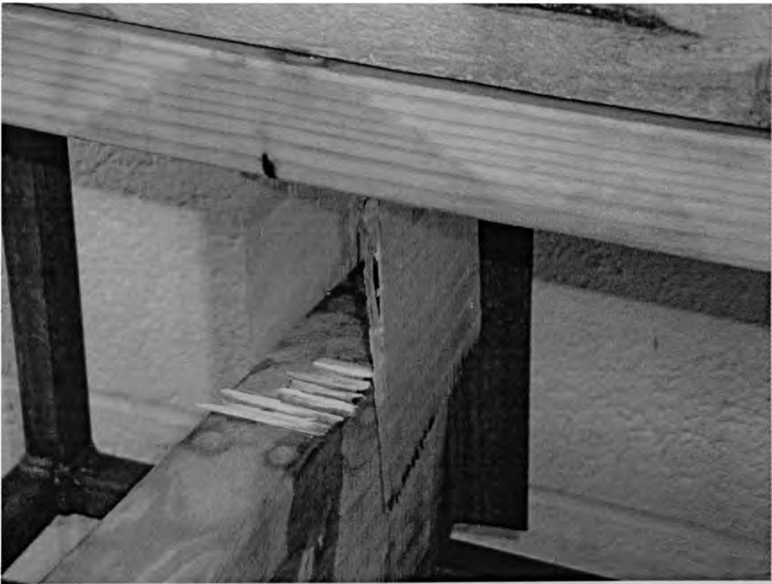
Figure 3.27 – Shear failure of specimen with longer FRP ties
