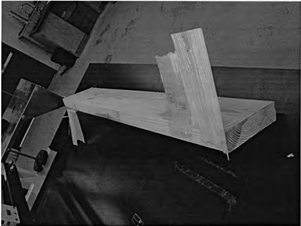
Figure 3.30 – Joist separating from top plates with FRP ties peeled off
