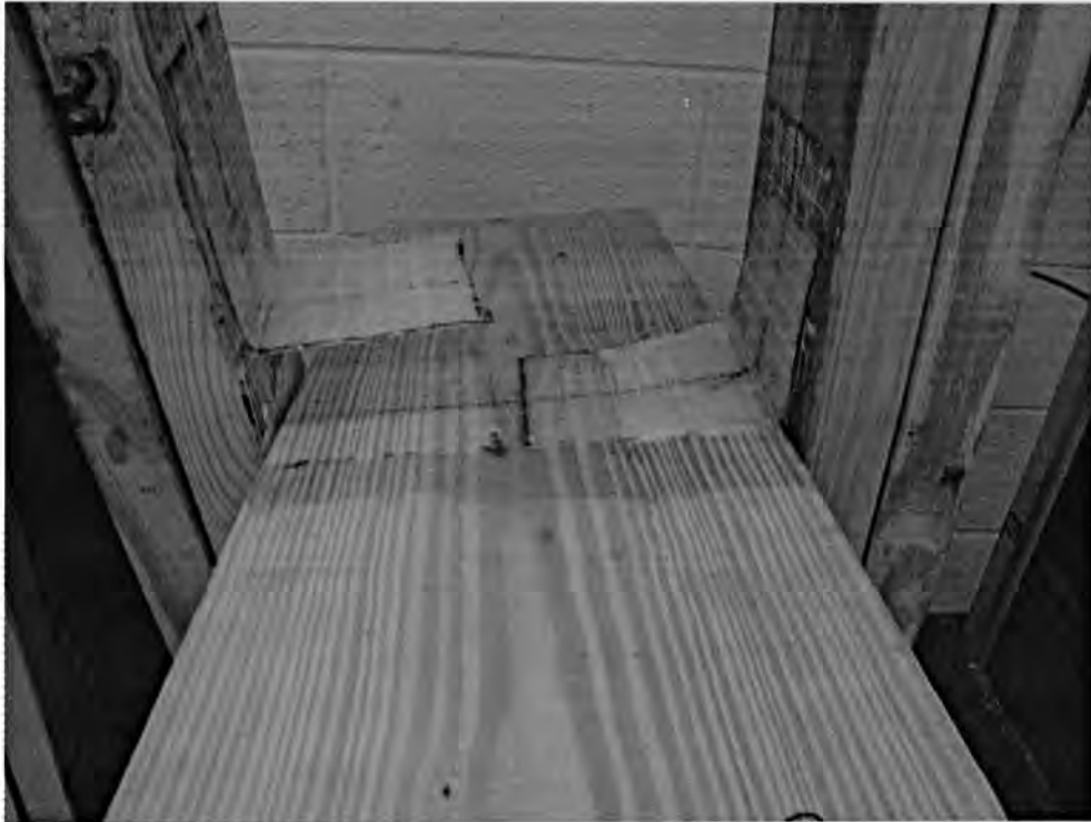
Figure 3.35 – Typical mode of failure under lateral loading
