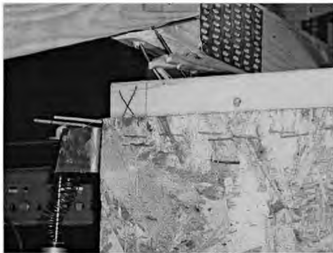
Figure 2.4 –Failed toe-nailed connection NISTIR 6938 by Riley and Sadek, 2003)
