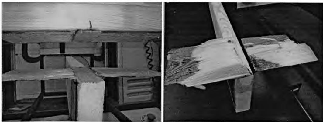
Figure 3.19 – Failure of Configurations A with GFRP (left) and CFRP (right)
