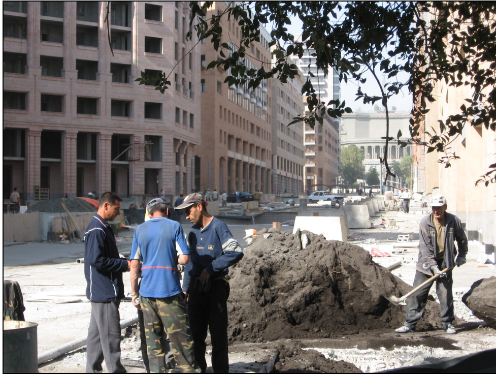
Figure 5.7: Northern Avenue, close to completion
