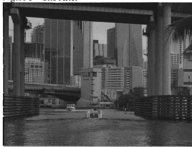
Figure 8 – Site Photo – Miami River
