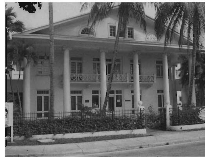
Figure 4 – Site Photo – Low Density Example
