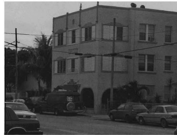
Figure 6 – Site Photo - Medium Density Example
