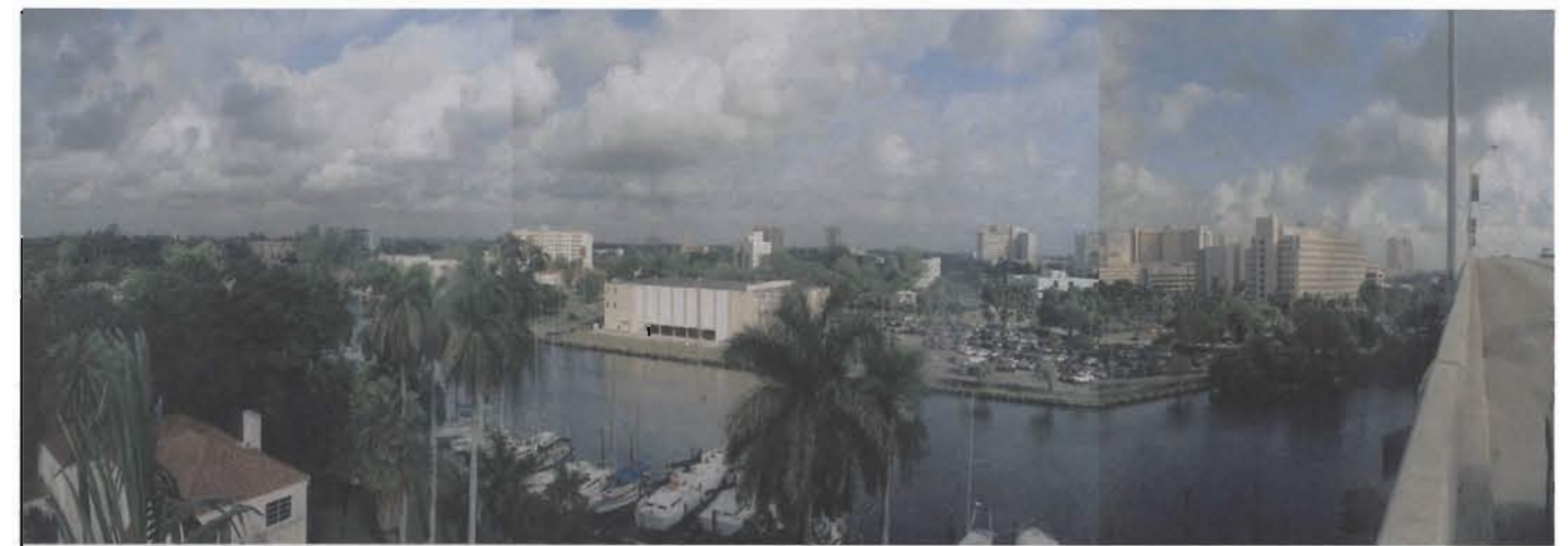
Fig.21 Intersection of Miami River and 836 Expressway (looking east).
