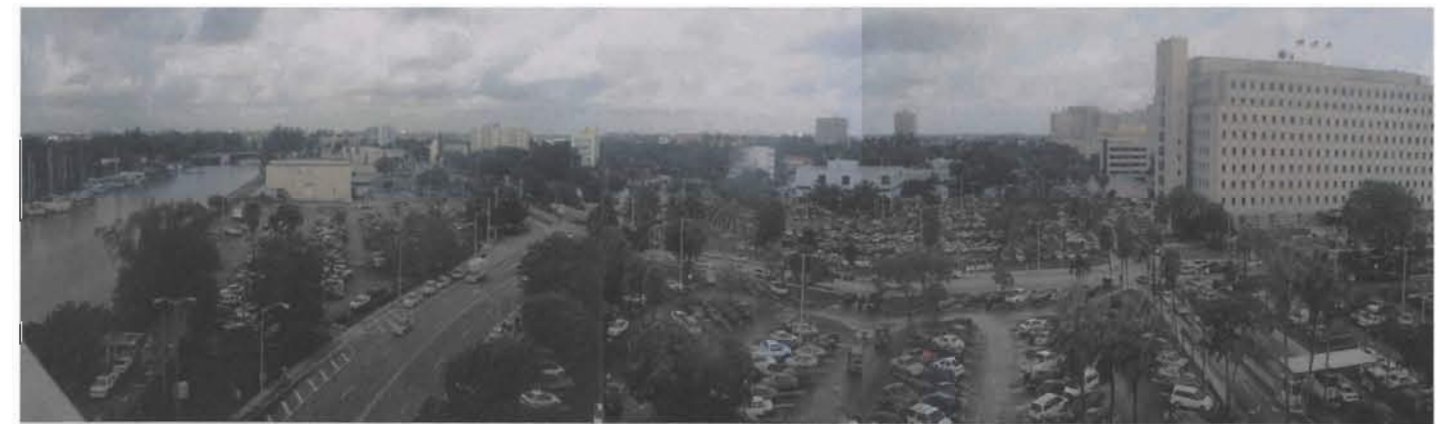
Fig.22 Intersection of Miami River and 836 Expressway (looking northwest).
