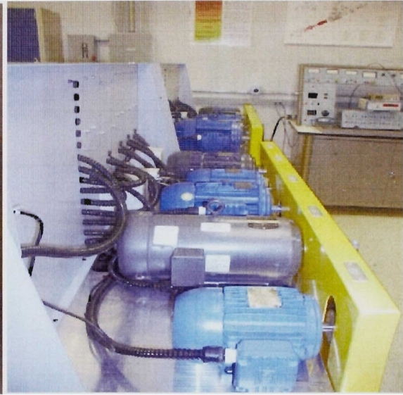
Figure 3.1-2 Generating station side view
