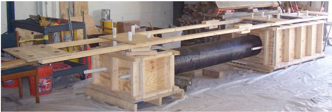
Figure 3.10 Template and Formwork for Specimen LC
