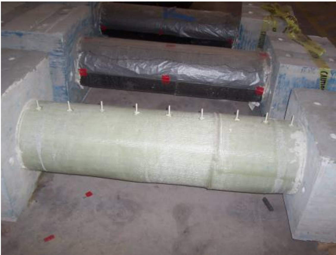
Figure 3.17 Port Layout for Epoxy Injection
