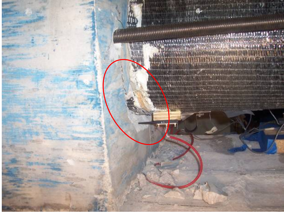
Figure 3.36 Concrete Spalling in Footing of Specimen H
