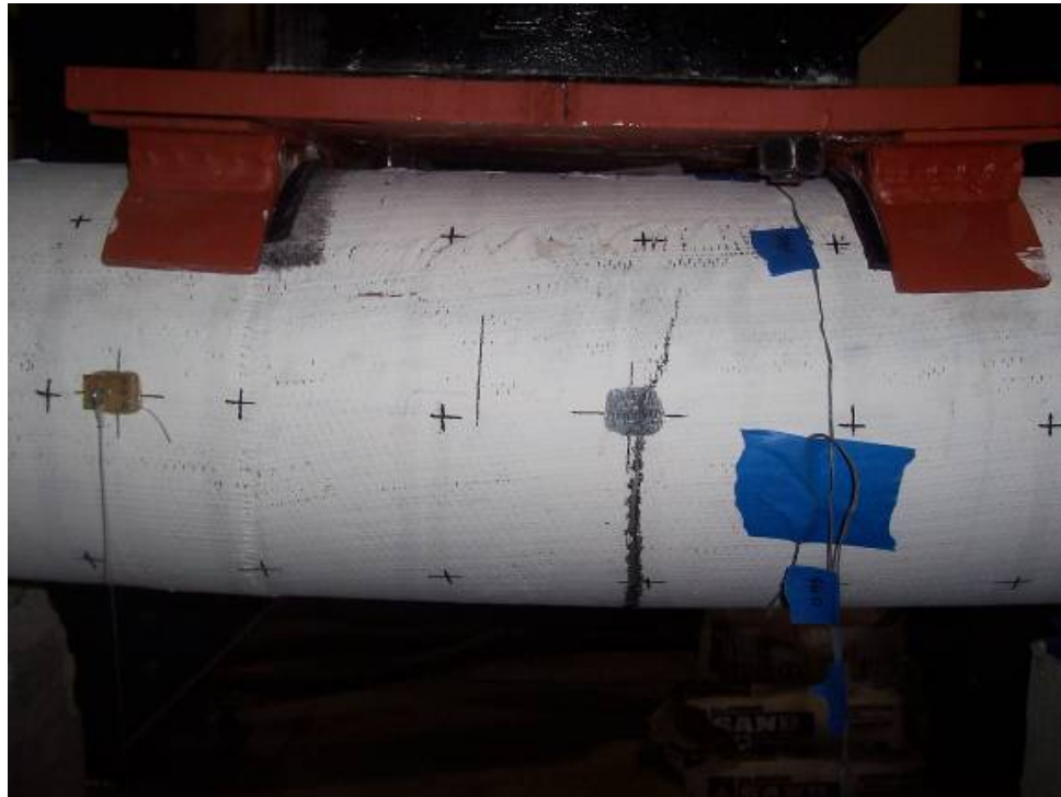
Figure 4.24 Flexural Crack in Specimen SC (West View)
