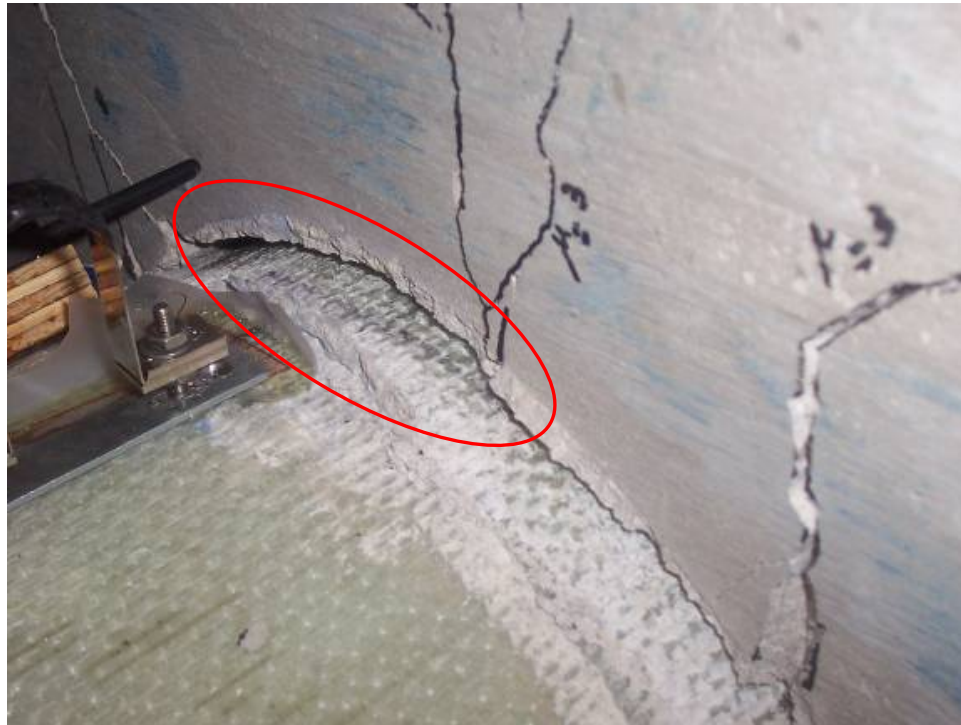
Figure 3.41 Tube Slippage in Specimen G
