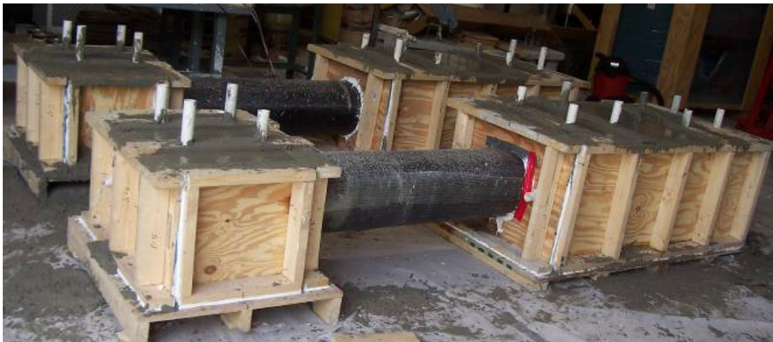
Figure 3.12 Specimens H and SC Right after Concrete Casting
