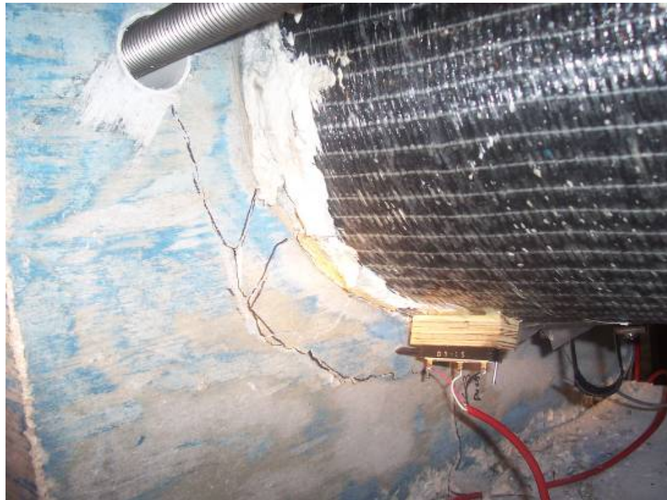
Figure 3.39 Splitting of Concrete Footing in Specimen H
