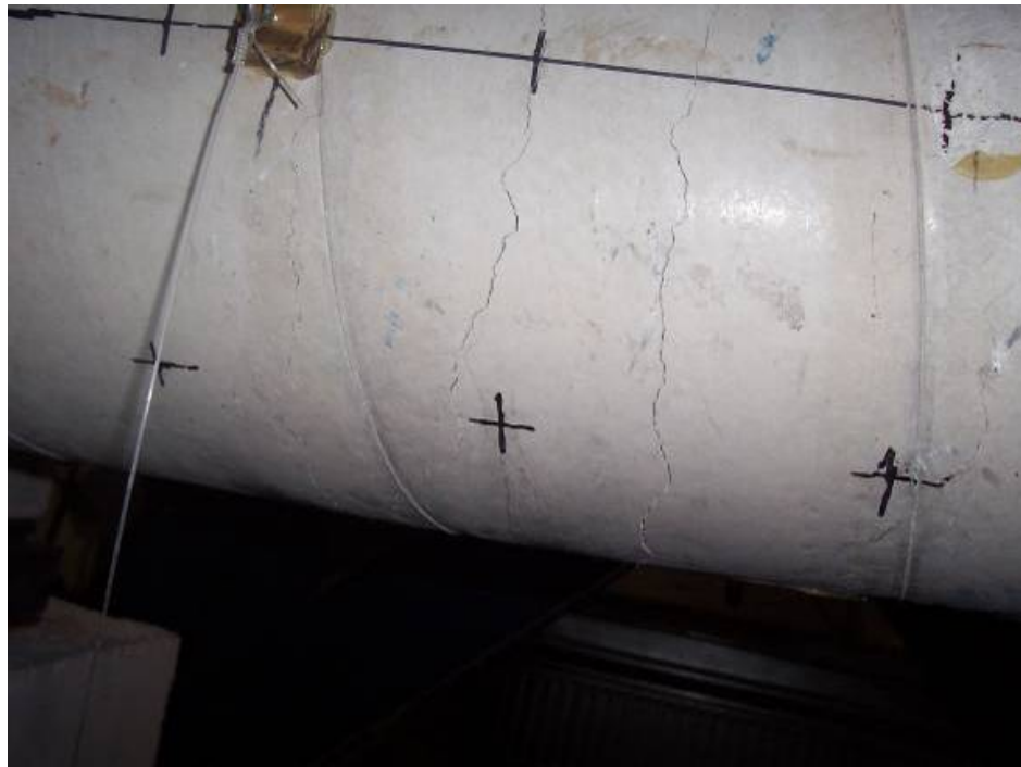
Figure 4.10 Flexural Cracks of Specimen RC at Mid-Span
