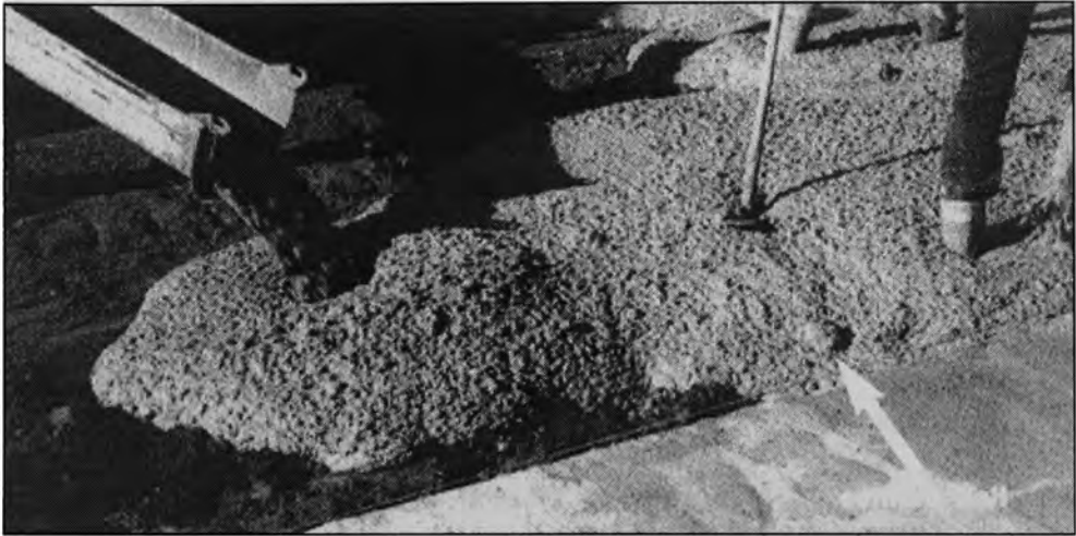
Figure 1.1 Concrete in Formwork (Gaynor, 1996)
