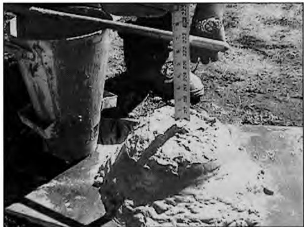
Figure 2.1 Slump of Concrete
