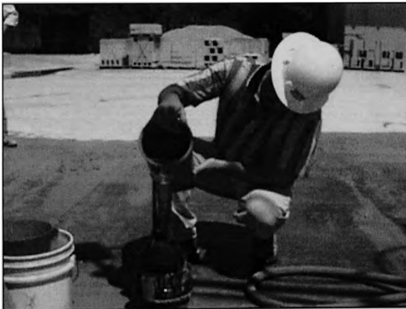
Figure 3.4 Concrete Air Content Test
