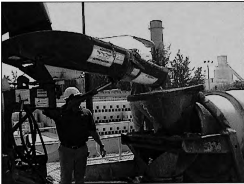
Figure 3.6 Discharging Concrete into Secondary Truck
