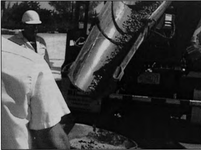
Figure 3.1 Concrete for Samples
