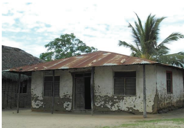
House roofed with iron sheets
