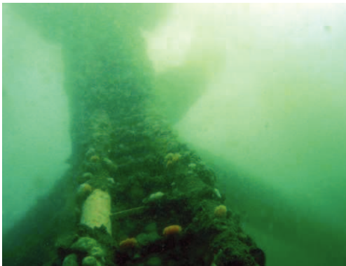
Fig. 6. the upper part of the offshore jacket foundation FINO1 (North Sea), densely colonized by epifauna (biofouling). (photo: Krone).
