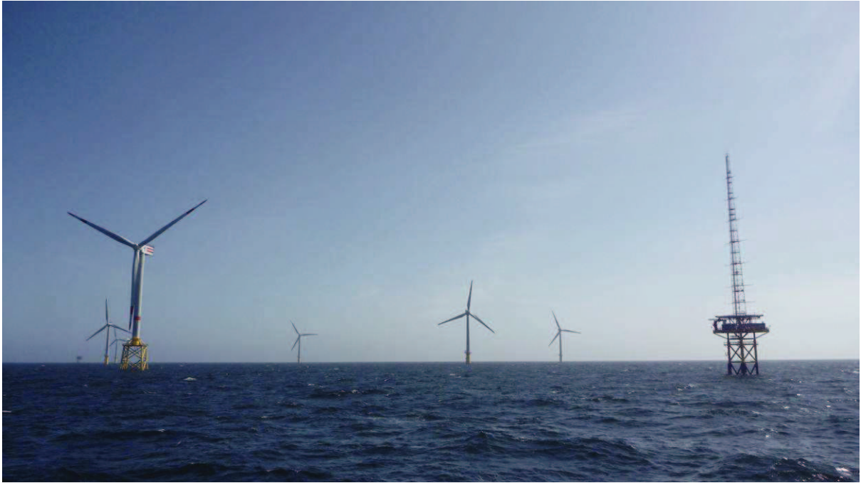
Fig. 5. The operating offshore wind farm alpha ventus 20 nautical miles northerly of the island of Borkum (North Sea, German Bight). Jacket constructions: research platform FINO 1 (right side) and wind power foundation (left side). Also other foundations are employed (the piles in the background) (photo: Krone).
