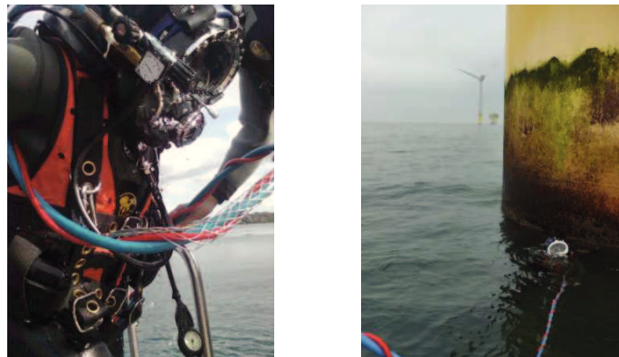
Fig. 10. Surface supplied diving equipment and diving at a large wind power pile at the wind farm alpha ventus , North Sea (photo l: Kanstinger, photo r: Krone).
