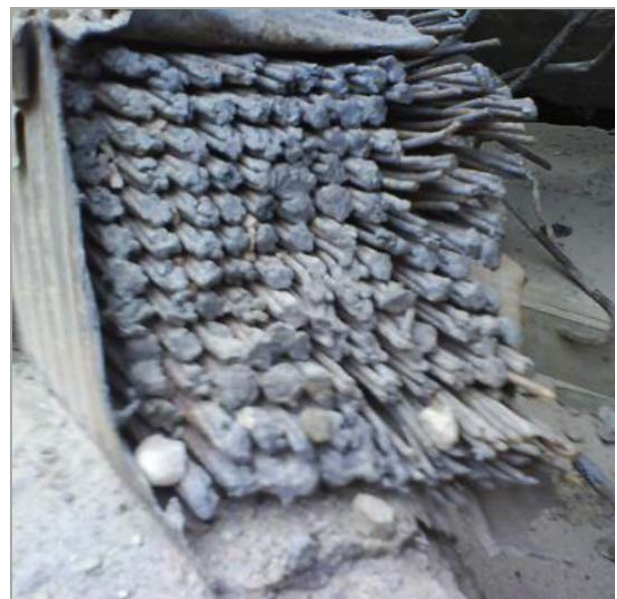
Figure 3. Opened tendon after demolition [15]
