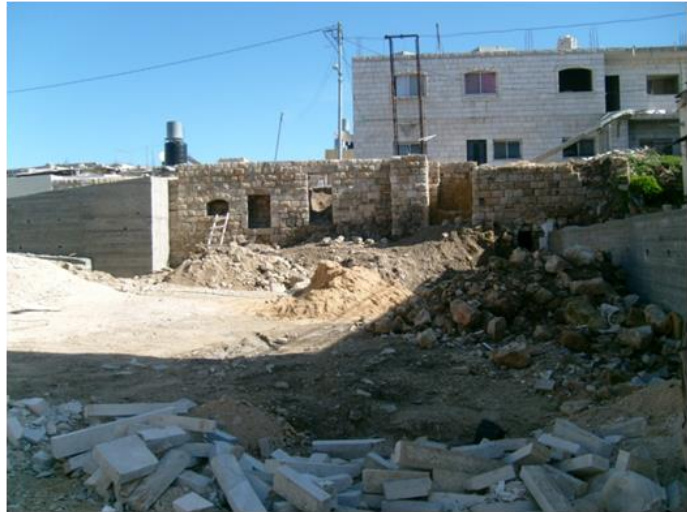
Picture 8-3: New modern buildings appear in the traditional quarter
